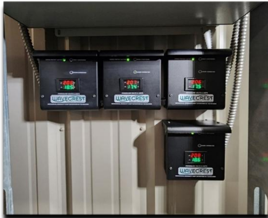
Figure 8: 208v LEDs was a unique aspect of this job
