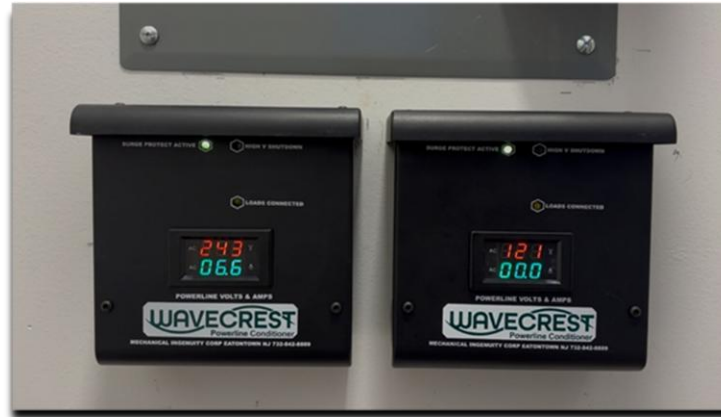
Figure 2: 240v & 120v units installed below the panel. Wavecrest can be mounted wherever is easiest for the installer.
